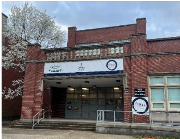
Pictured: Neighborhood Place Northwest
